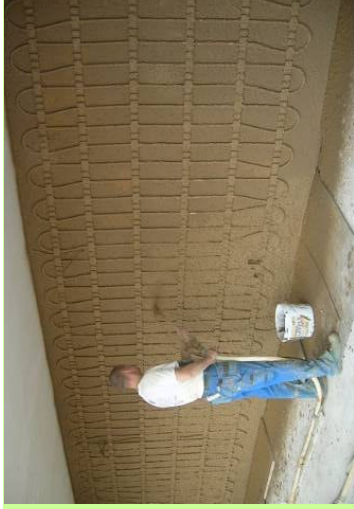
Applying the clay plaster
