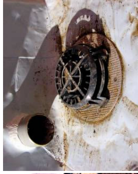
Detail of the EPDM liner over the cork insulation
