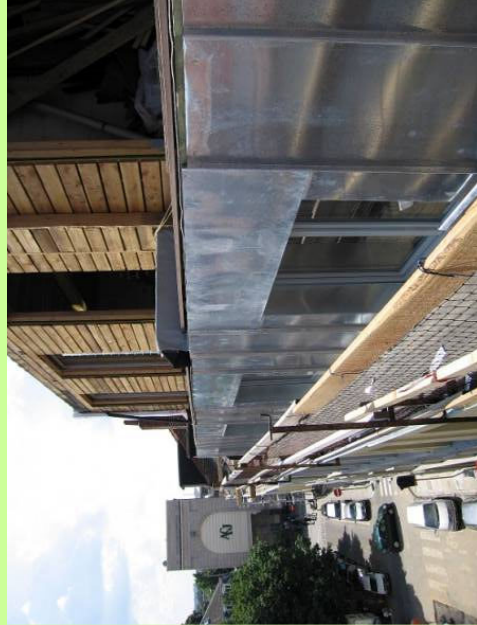
View on the terraces of the triplexes and duplexes, North side. Part of the wall already has a zinc finishing.
