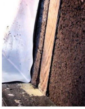
Detail of the EPDM liner over the cork insulation
