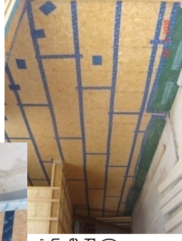
Taping off the OSB boards, and connection between OSB and plaster on the brick walls (the white band in the upper photo)
