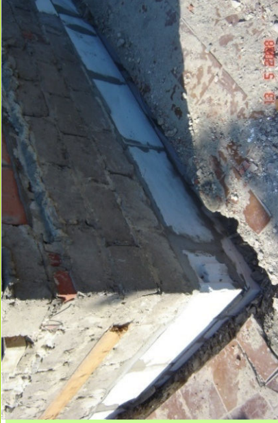
Thermal break at the base of the walls
