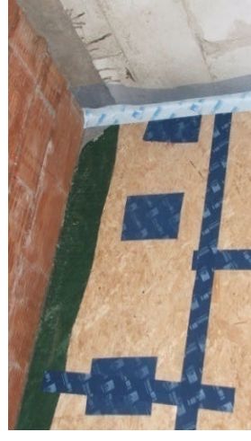
Taping off the OSB boards, and connection between OSB and plaster on the brick walls (the white band in the upper photo)
