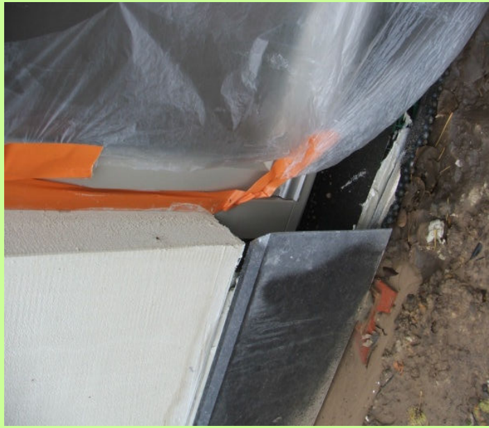
Connection threshold with front floor.
