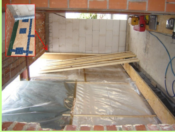
The construction of the common wall
