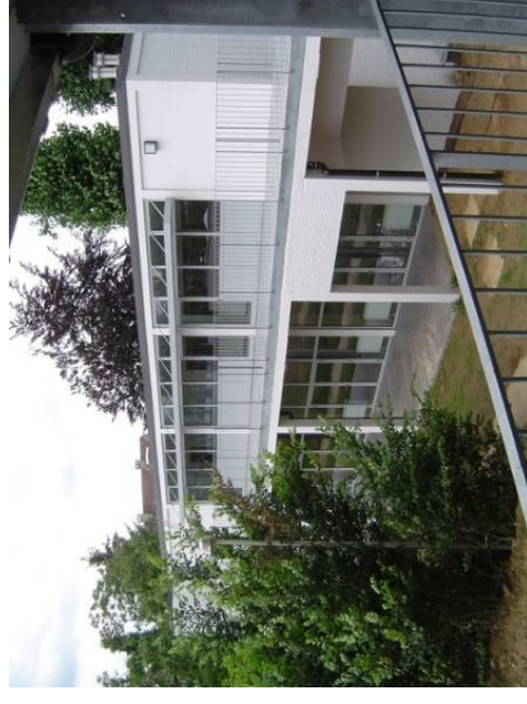
The old co heating boiler room, now a community centre and small office block.
