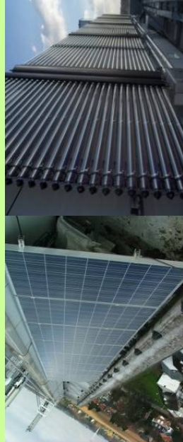
photovoltaic solar panels and vacuum tube solar heating system on the roof of Sterrenveld.
